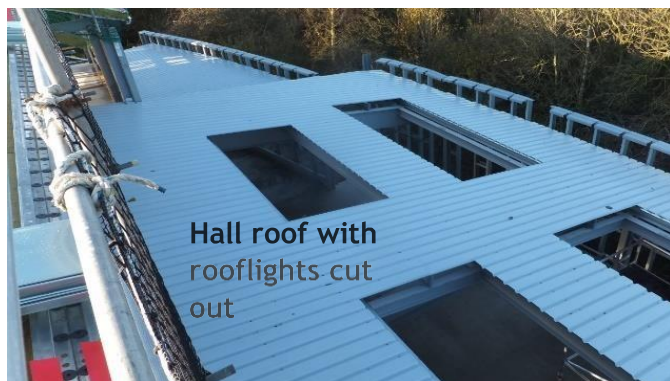
Rooflight kerbs ready to take horizontal windows
