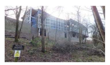
The timber lining to the first floor is complete and the metal gutters are also now fixed.
