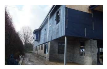
If you have driven past recently you will have seen a lot of blue! This is the breathable membrane which prevents moisture affecting the inner walls and will shortly begin to be concealed behind a combination of metal cladding, larch boarding and coloured render.
