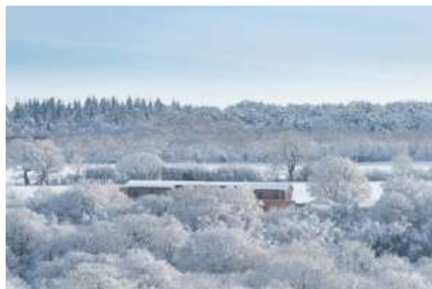
Thank you to Tim Hardy Photography for these brilliant drone shots of the new Birk Crag Centre.
