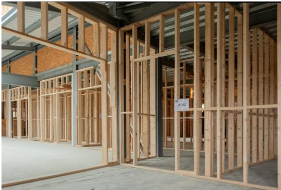
The ground floor and first floor wall studding is almost complete.
