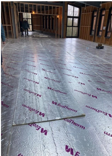
The ground floor underfloor heating is being installed this week!
