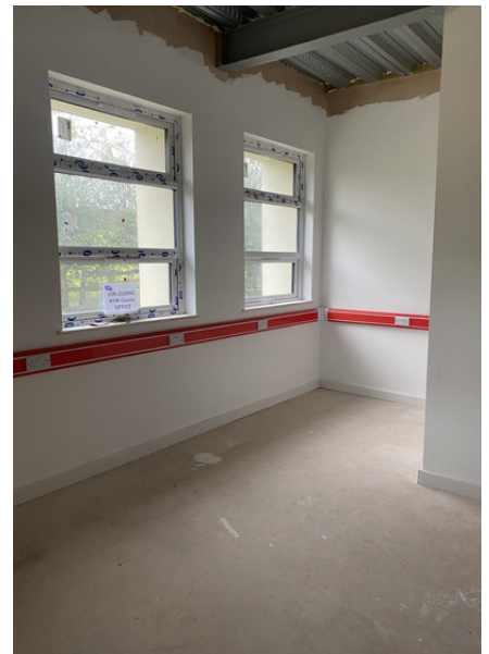
Our NYW County Office taking shape
